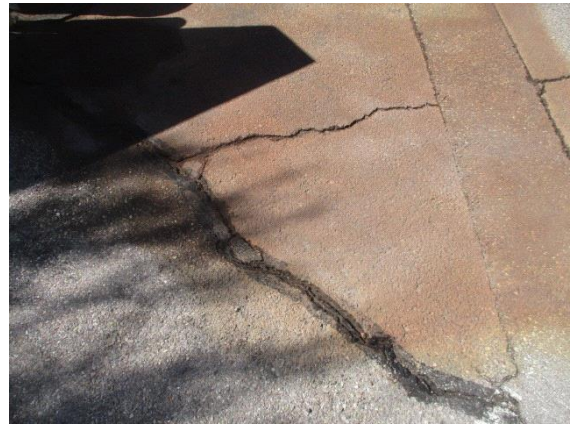
Parking Lot / Driveways:
