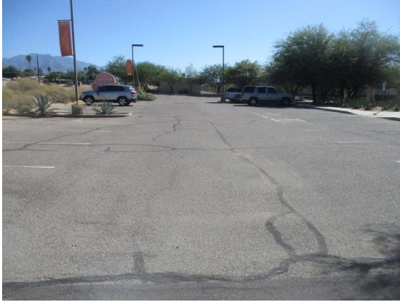
Parking Lot / Driveways:
