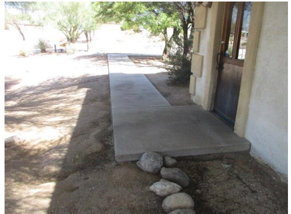
Flatwork / Sidewalks: Ground Should Be Built Up
