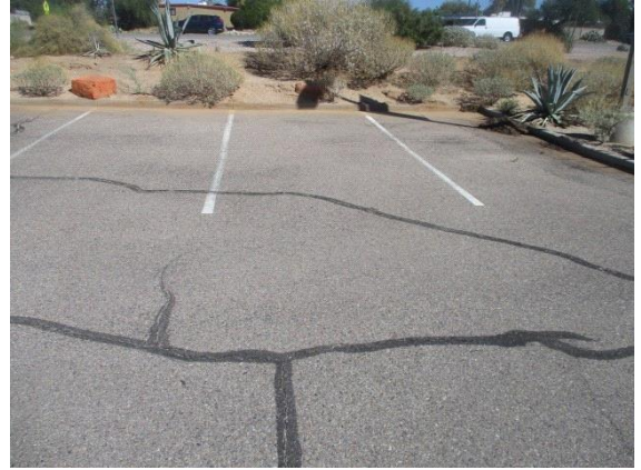
Parking Lot / Driveways:
