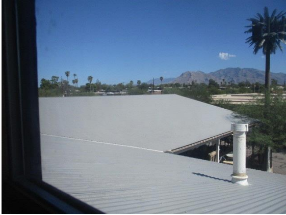
Roofing: Southeast Roof
