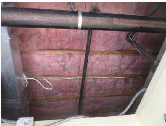
Structural Frame and Building Envelope:
