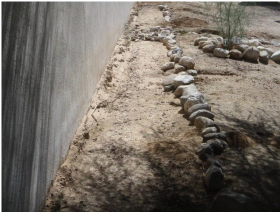
Grading / Drainage: West
