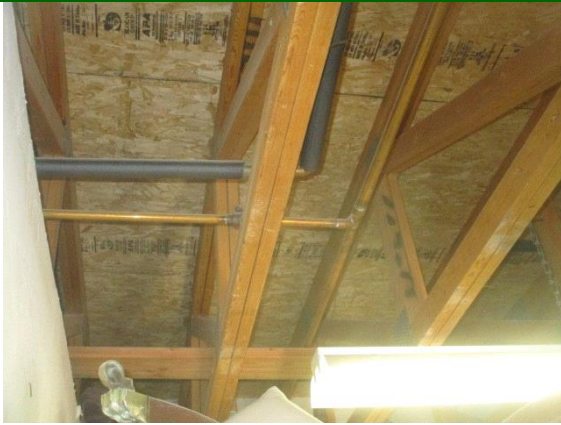
Structural Frame and Building Envelope:
