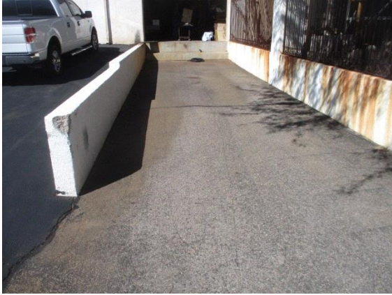
Parking Lot / Driveways:
