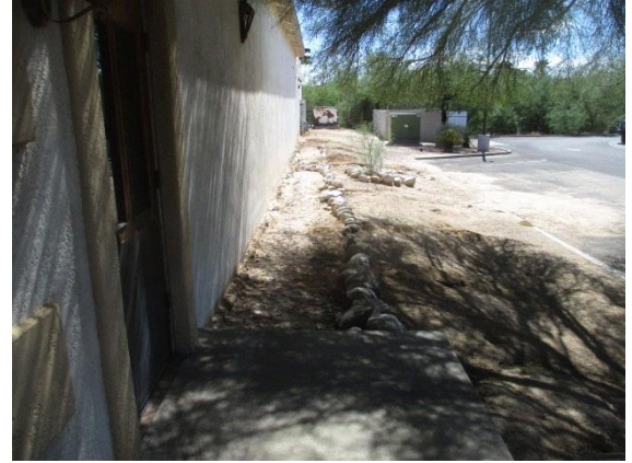
Grading / Drainage: West
