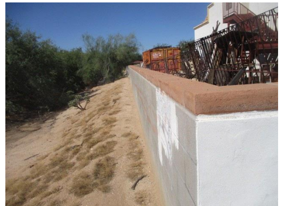
Grading / Drainage: Rear(South)
