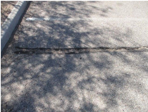
Parking Lot / Driveways:
