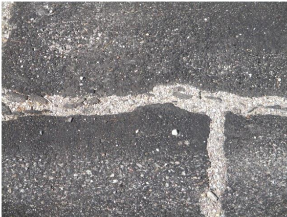
Parking Lot / Driveways:
