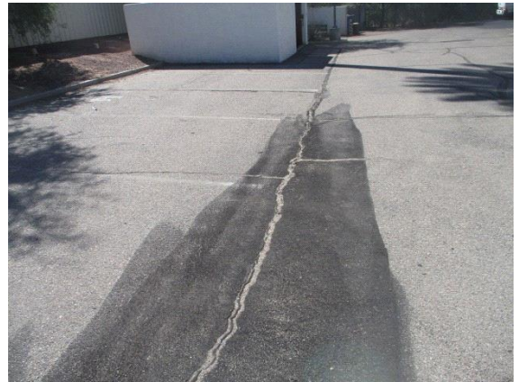
Parking Lot / Driveways:
