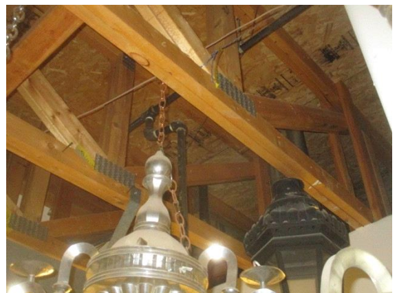
Structural Frame and Building Envelope:
