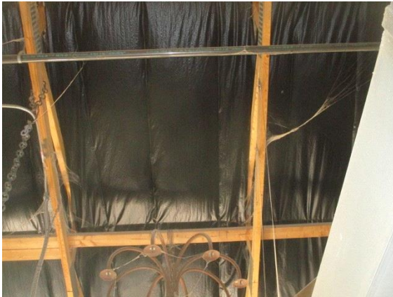
Attic / Roof Framing and Sheathing:
