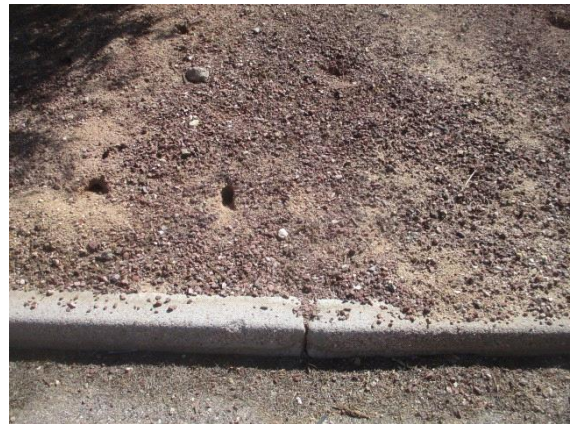
Landscaping: Holes In Ground
